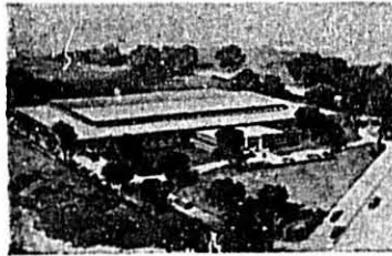
This is architect's drawing of the new $500,000 plant which will house Modern Packages, Inc., Memphis subsidiary of American Coating Mills, Elkhart, Indiana. It is expected that the new buildings will be ready for occupancy about March 1.
